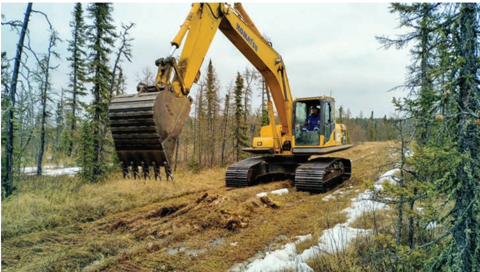
Figure 2A. Low ground disturbance tracked excavator.
