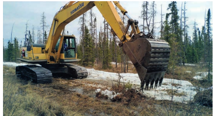
Figure 3D. Placing intact hummock.
