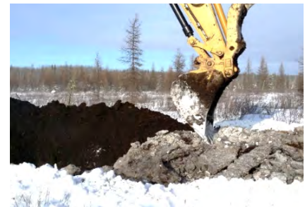
Figure 3. Stripping chips and piling of peat using a backhoe.
