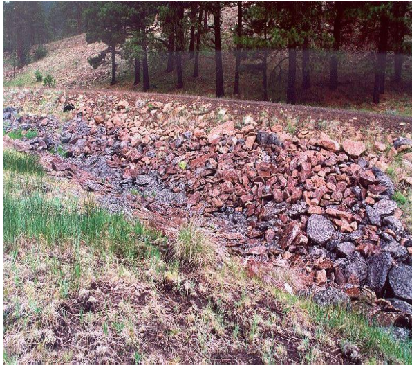
Figure 10. Cobble armour used to prevent erosion along a road cut (USDA-Forest Service image)
