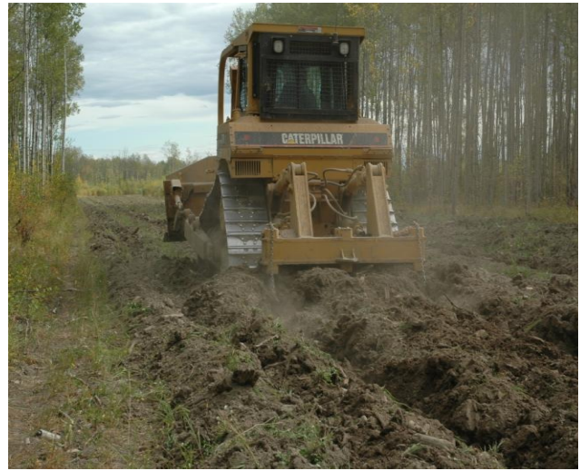
Figure 12. Using Rip-Plows® to de-compact a road.
