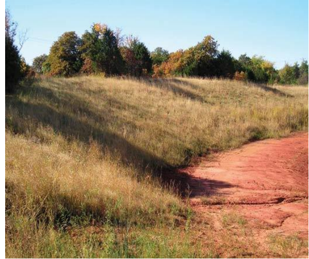
Figure 7. Result of using erosion netting on an erodible side slope.
