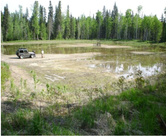
Figure 11. Water ponding on the surface of a compacted well site.
