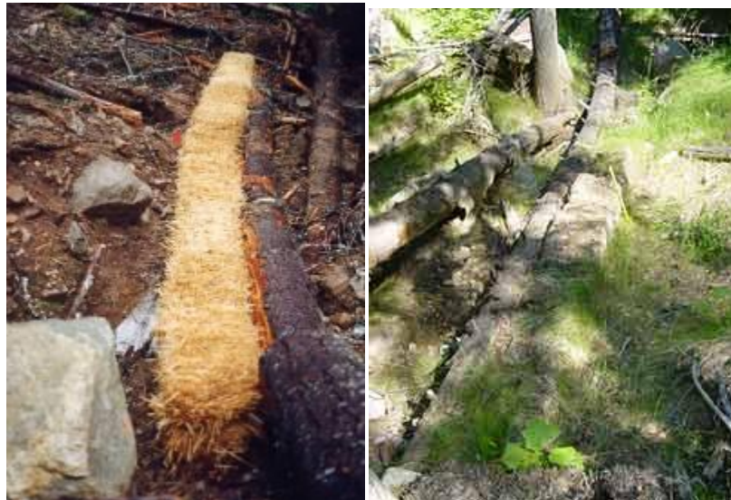
Figure 8. Straw bale erosion control at install and 6 years later.
