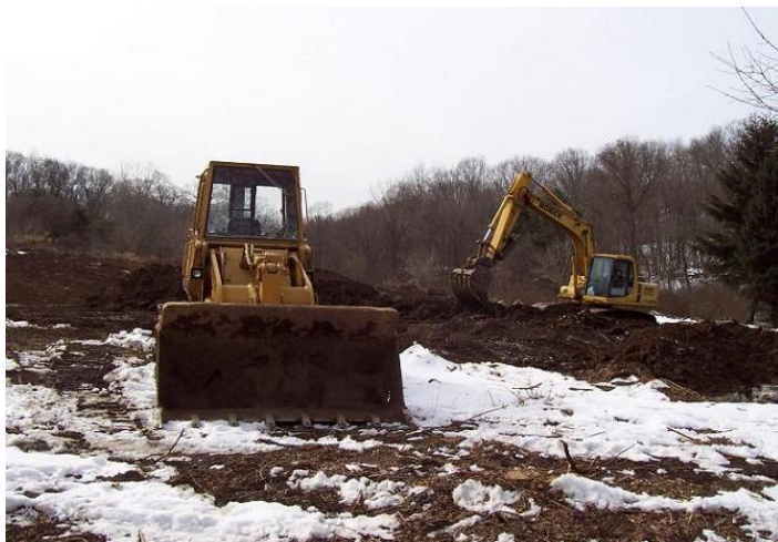
Figure 15. Dozer and industrial backhoe salvaging topsoil (note storage piles).
