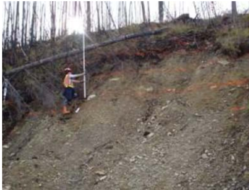
Figure B-48 Slope failure at Beaver Creek within the pipeline right-of way.
