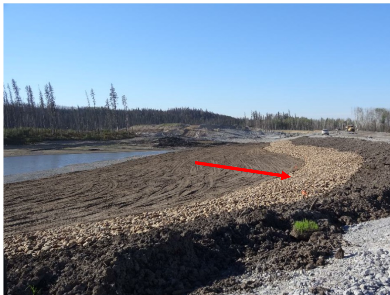
Figure B-41 Riprap armouring along the shoreline of the compensation lake.
