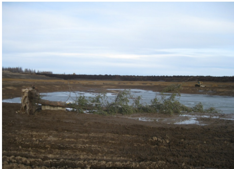
Figure B-47 Coarse woody material used to provide fish habitat in compensation lake.
