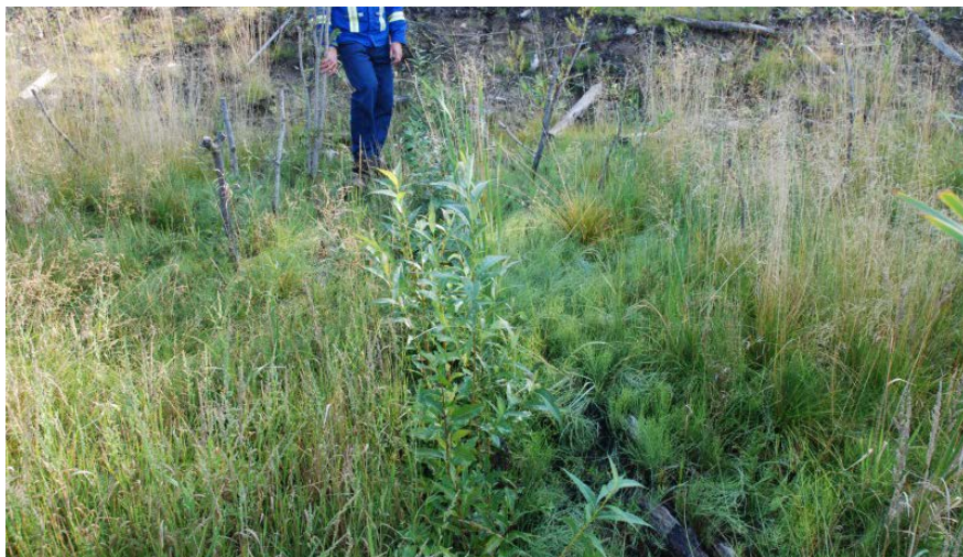
Figure B-8 Live pole drains used to reduce excess water that had lead to slope failure (August 27, 2012).
