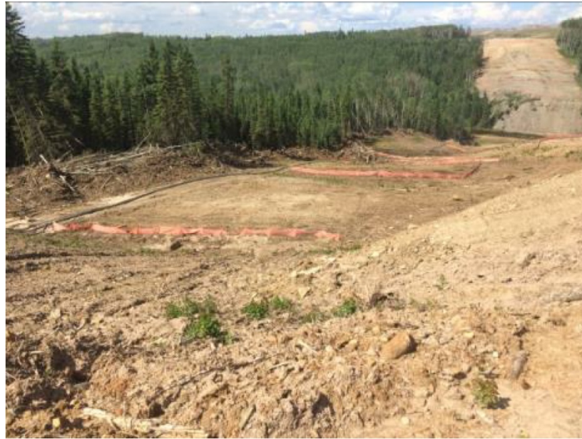
Figure B-33 Silt fences used for on-lease fire breaks at Base Mine.
