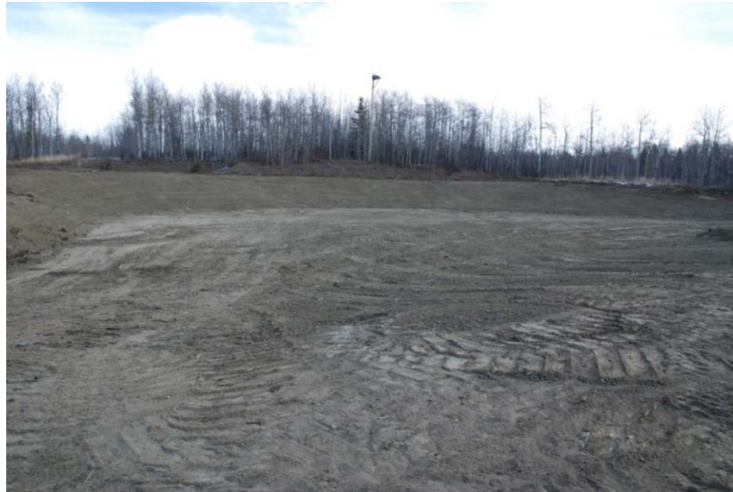
Figure B-91 Exposed soil at the gas plant was decontaminated and regraded (compacted and smooth).
