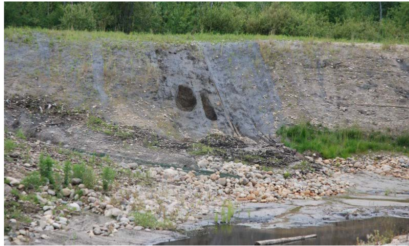
Figure B-5 Slump under erosion control matting.
