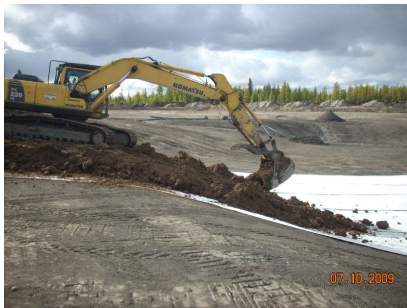
Figure B-45 Cover material application over the geosynthetic clay liner in compensation lake.
