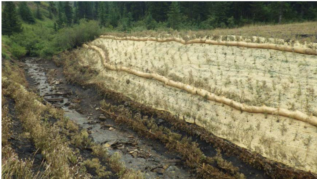
Figure B-69 Coconut matting and straw logs installed to protect exposed soils along the McLeod River.
