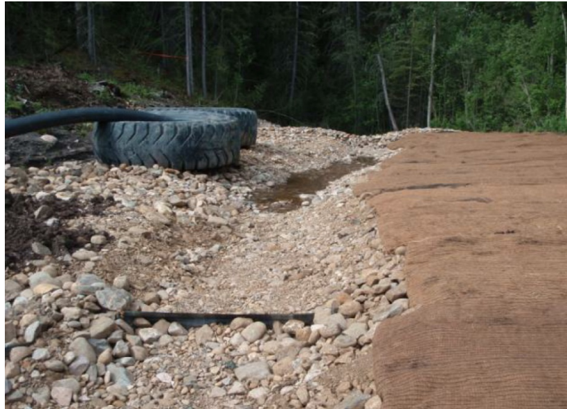
Figure B-46 Outlet channel at compensation lake lined with cobbles and coconut matting.
