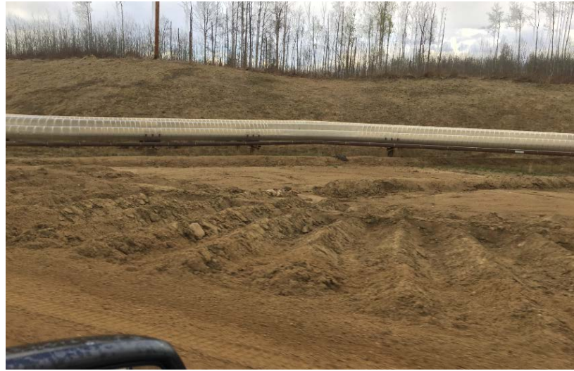
Figure B-14 Soil check dams adjacent to pipeline corridor and a road.
