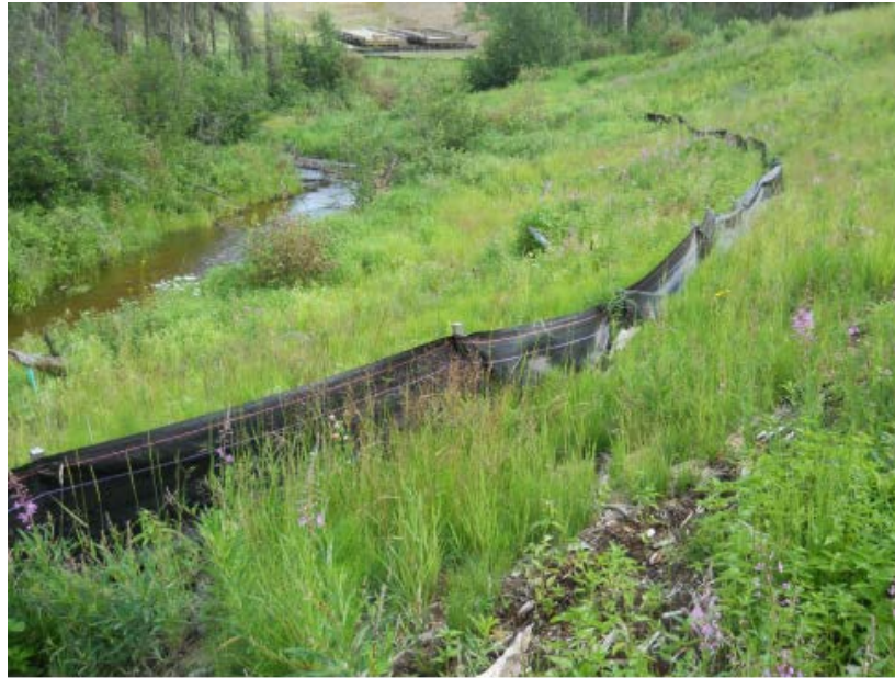
Figure B-35 Silt fence and revegetation near Clarke Creek.
