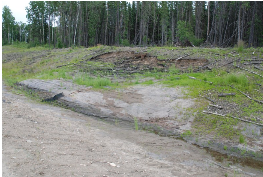
Figure B-6 Slumping and erosion control mat failure along the east side.
