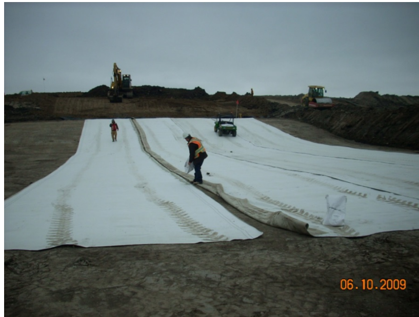
Figure B-44 Installation of the geosynthetic liner in compensation lake with a 12-inch overlap between sheets.
