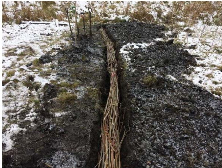
Figure B-28 Live fascines that have been placed in the 30 cm by 30 cm trench.
