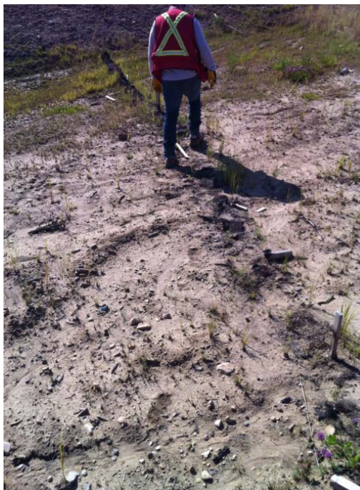
Figure B-36 A silt fence burnt by 2016 fire. Remaining soils have poor vegetation cover.
