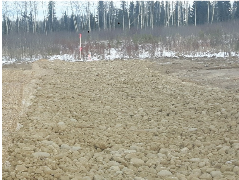
Figure B-24 An armoured drainway releasing into vegetated areas at Kinosis Borrow Pit.
