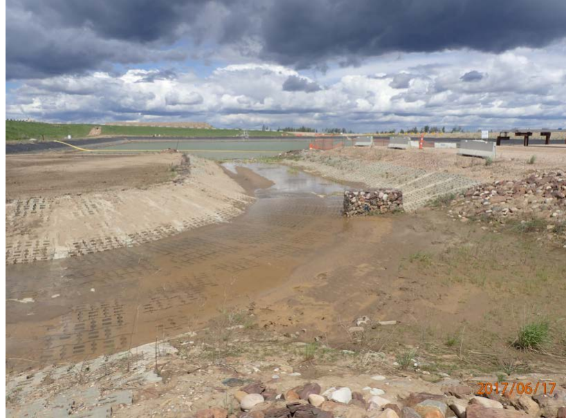
Figure B-15 Spillway at CPF illustrating the various conventional ESC measures used to manage erosion.
