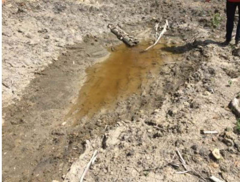
Figure B-32 Ponded water along fire breaks at Base Mine. Regrading to move water towards natural vegetation has been proposed.
