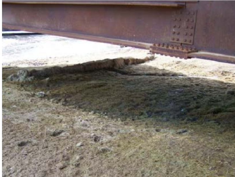
Figure B-83 Straw check-dams one year after installation.
