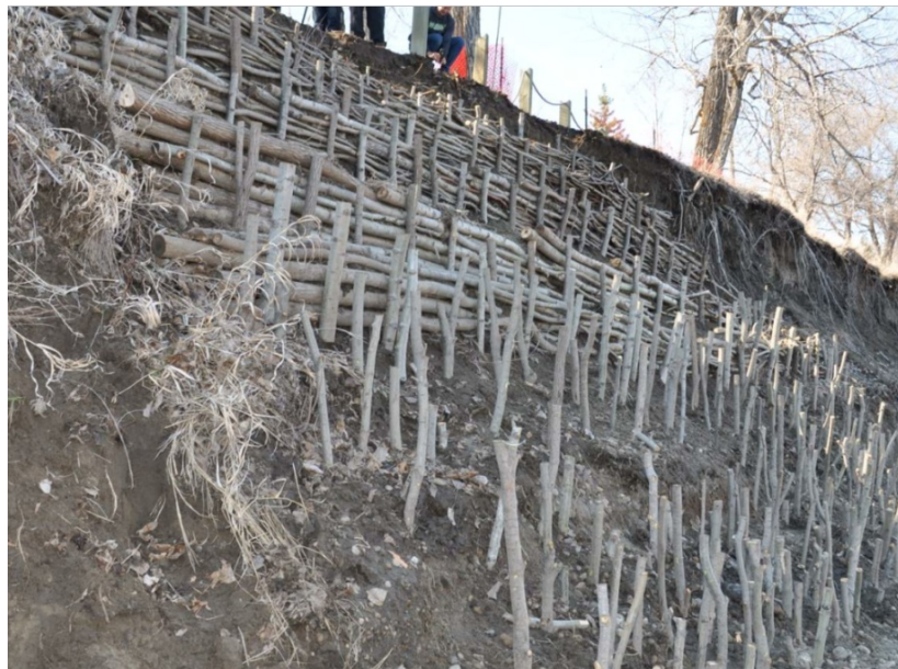
Figure B-86 The upper 75% of the slope was stabilized using wattle fences, the lower 25% using live staking (April 19 th , 2017).
