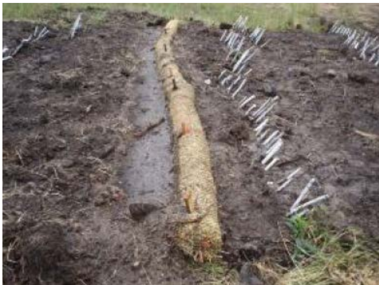
Figure B-55 Brush layers and straw coir rolls installed along slope in June 2006.
