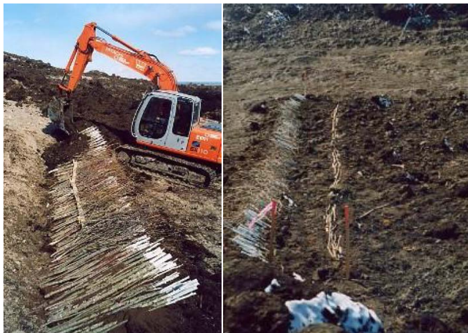
Figure B-61 Brush layering installation (left); live fascines used in combination with brush layering (right).
