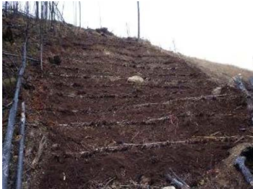
Figure B-49 Brush layers and live fascines installed on pipeline right-of-way, October 2004.
