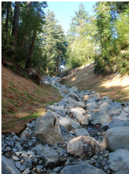
Figure B-77 Riprap was partially covered in soil, seeded with grass, and stabilized using coconut matting (2012).
