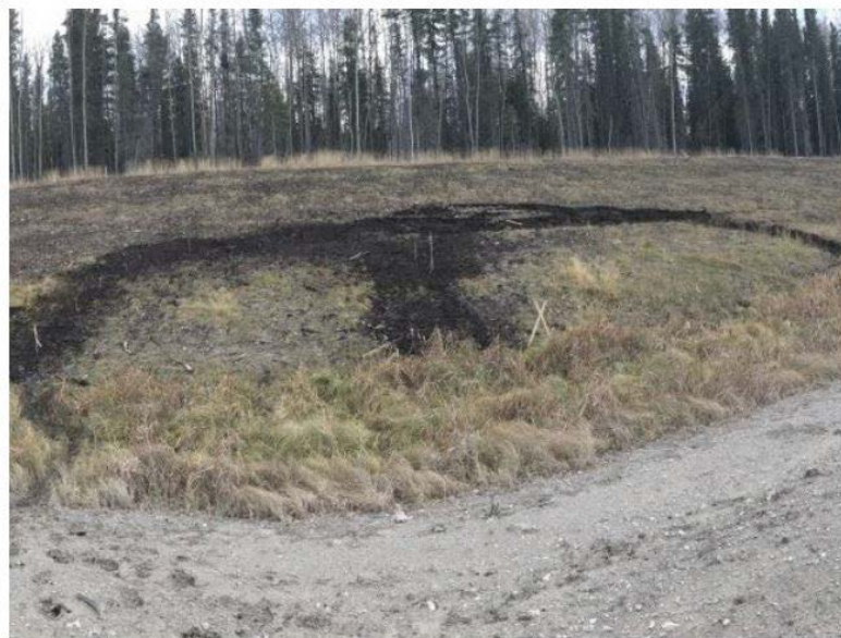
Figure B-29 The completed view of the arched "M" shaped live pole drain trench.
