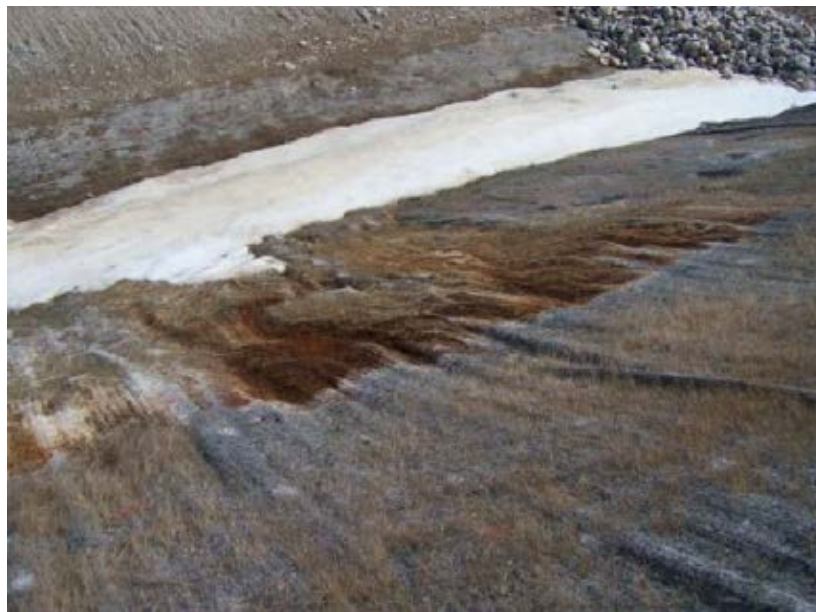
Figure B-84 Failing erosion control matting with minimal or no vegetation growth one year after installation.
