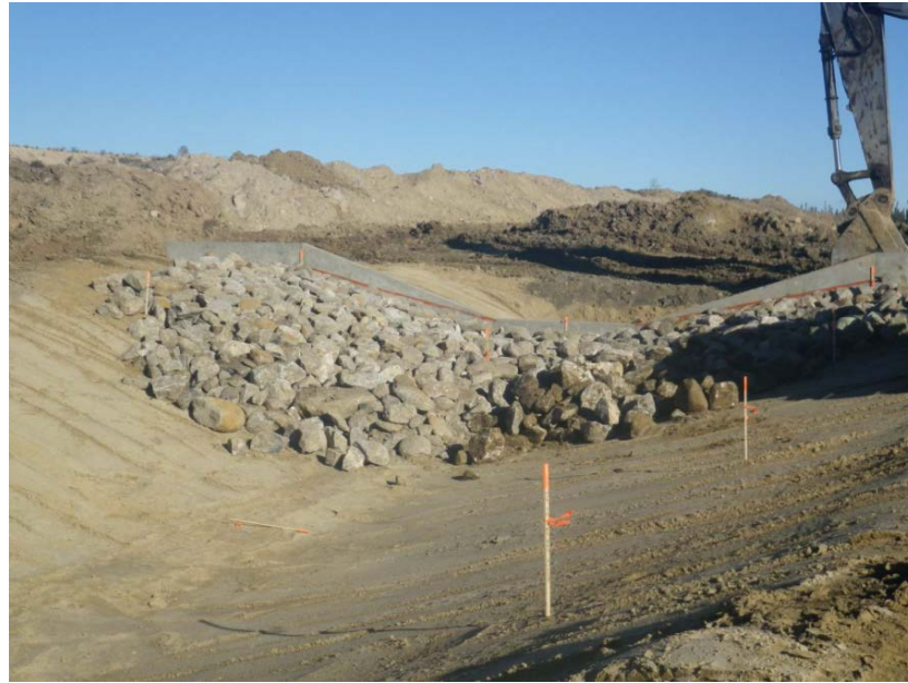
Figure B-31 Drop structure installed along a perimeter ditch with riprap armouring at MD9.
