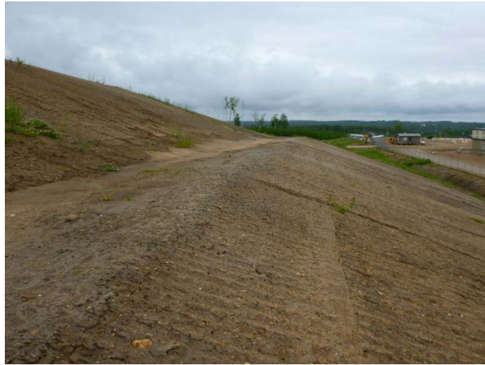
Figure B-22 Unsuccessful hydroseeding on a subsoil stockpile at Surmont.
