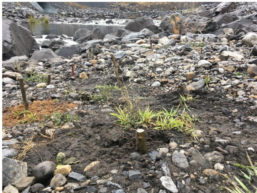
Figure B-73 Fording River after the live cuttings were planted in October 2017.
