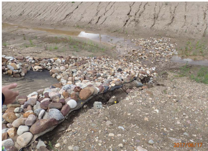
Figure B-18 Water bypassing the rock guards along the South Ditch.
