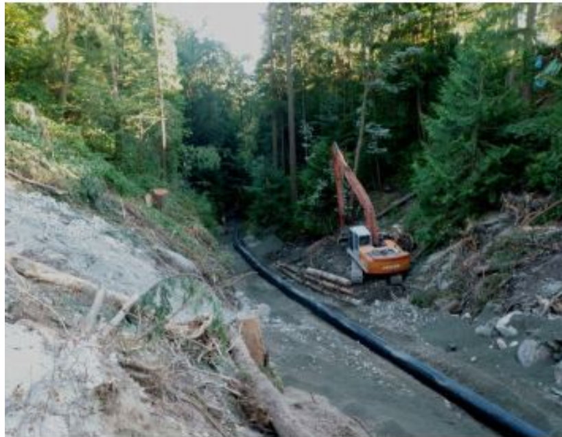
Figure B-78 Diversion pipe installation (2012).
