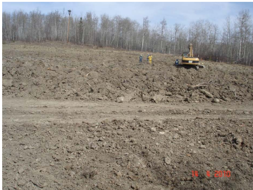
Figure B-92 Rough and loose soil treatment.
