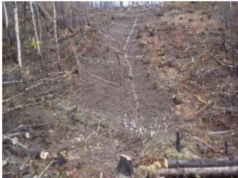
Figure B-52 Live pole drain installation at failure site, October 2005.
