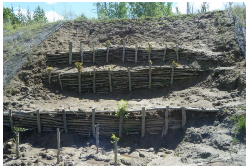
Figure B-2 Wattle fence installation after erosion control matting failed (June 27, 2012).
