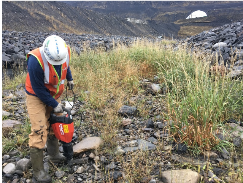
Figure B-72 Live cuttings were planted below the boulders.
