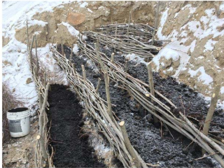
Figure B-30 The wattle fence backfilled with excess cuttings, live fascines, and peat.
