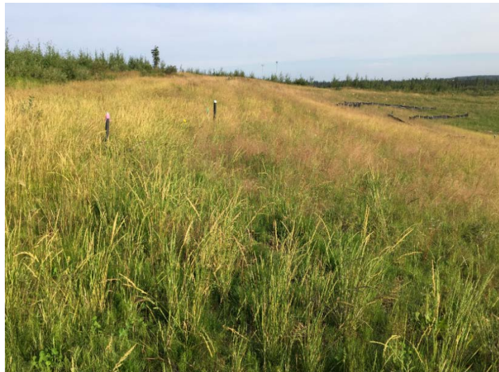
Figure B-21 Successful hydroseeding on a borrow pit at Surmont.
