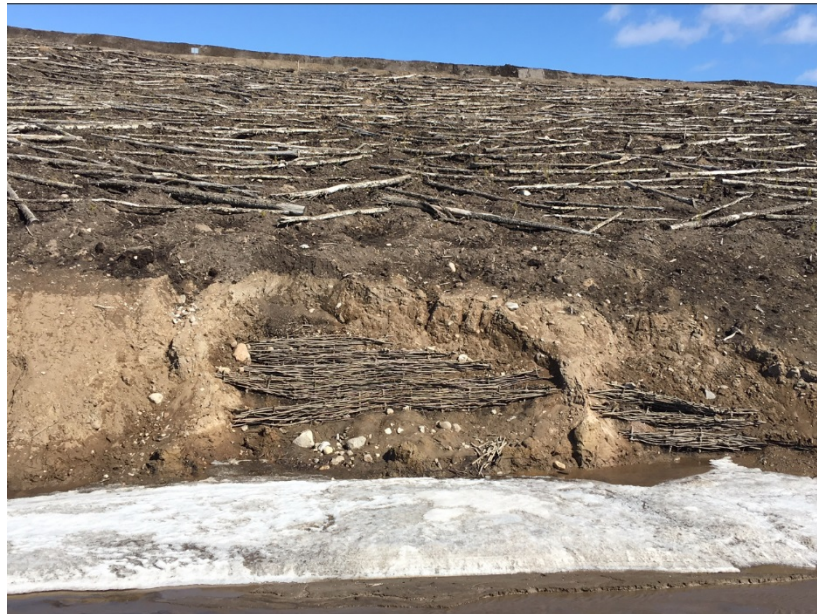
Figure B-29 Four-tiered wattle fence constructed along a 5:1 (11°) slope on overburden dump.
