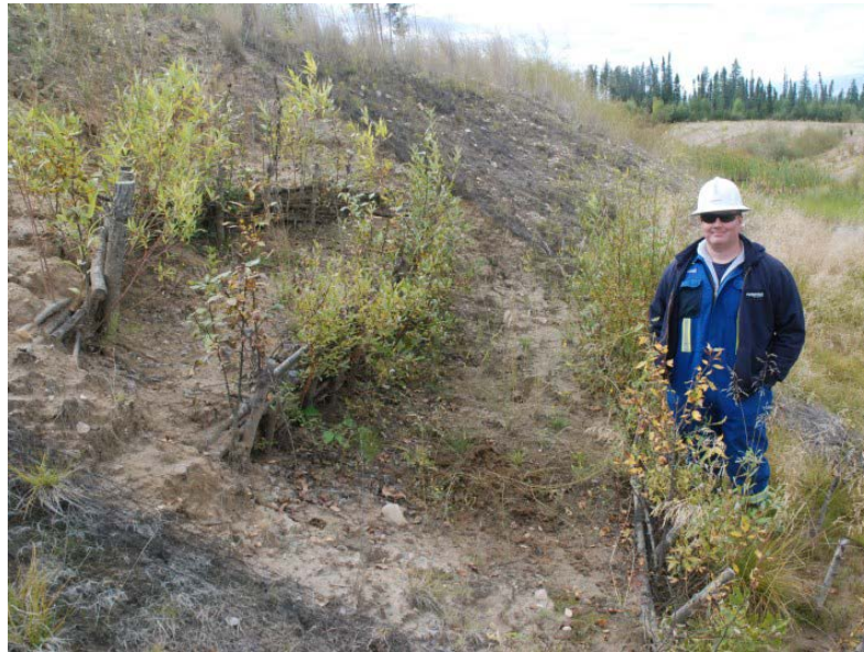
Figure B-3 Successful establishment of the wattle fence; growth two years after installation (September 10, 2014).
