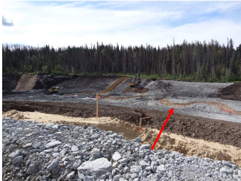
Figure B-40 Riprap armouring and soil placement along the outlet channel leading from the compensation lake.
