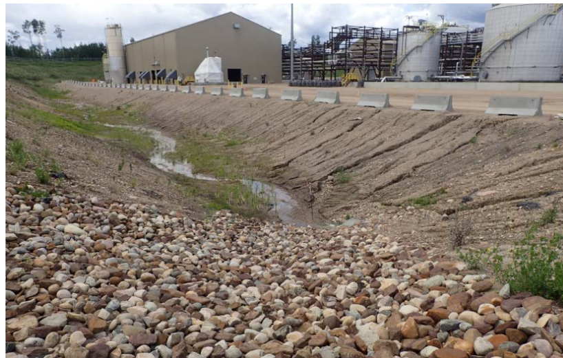
Figure B-16 CPF South Ditch rills.
