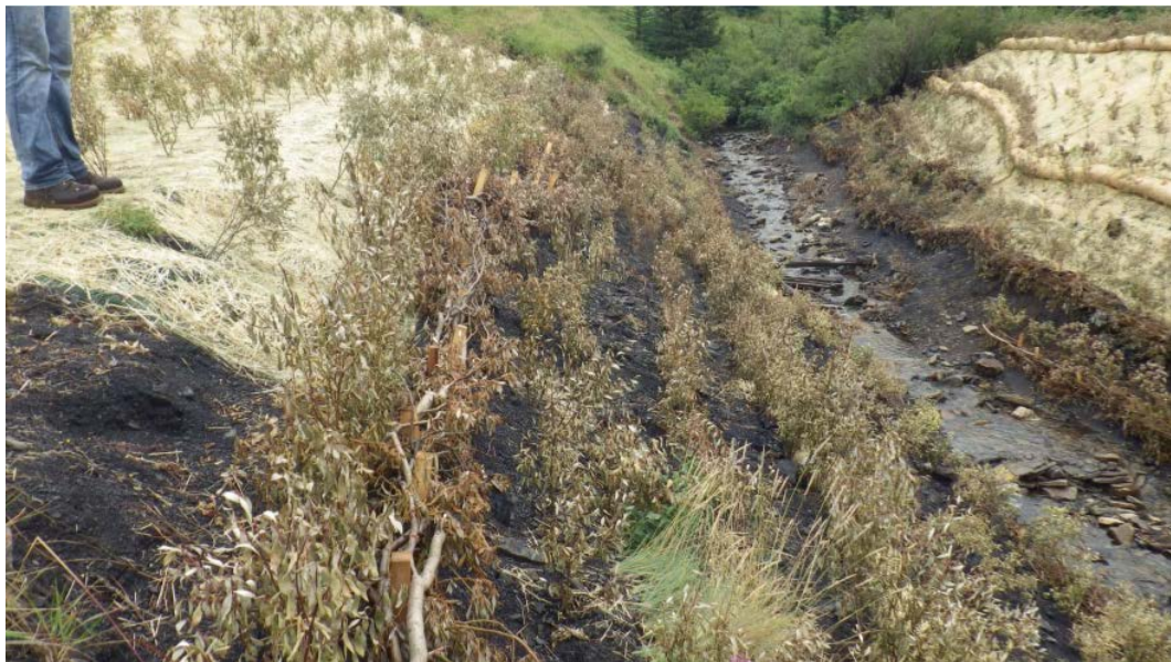
Figure B-70 Wattle fencing installed along a stream bank along the McLeod River.
