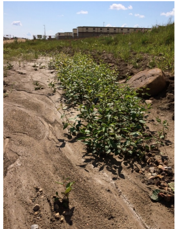
Figure B-20 Live staking survival and re-growth at Surmont.
