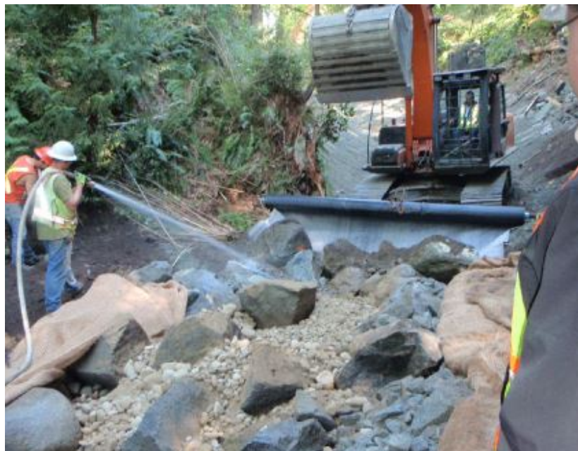
Figure B-79 Conventional techniques for ravine bed: geosynthetic liner, riprap, and large boulders (2012).
