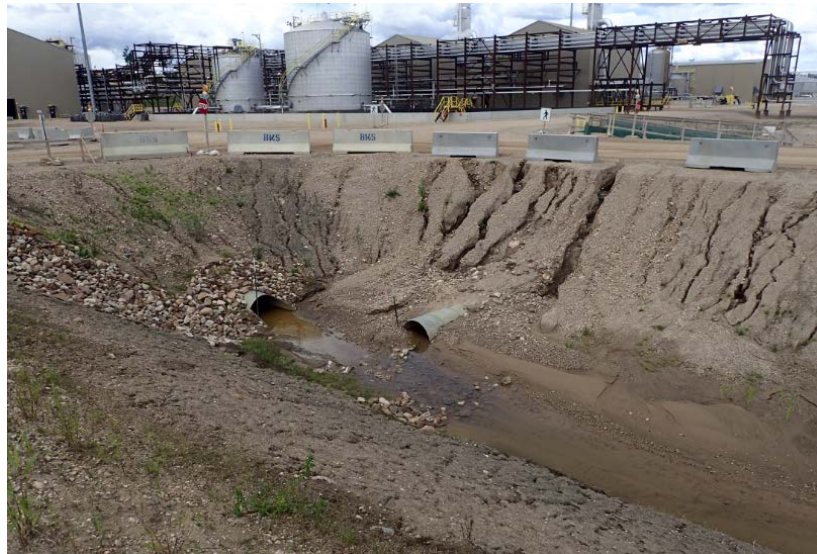
Figure B-17 CPF South Ditch rills.
