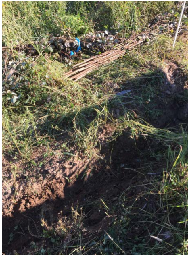
Figure B-19 Trench and live pole drain prior to installation at 12-24-083-06 W4M.
