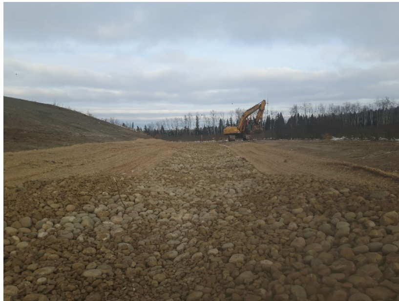
Figure B-23 Coconut matting with riprap armouring a drainway at the Kinosis Borrow Pit.
