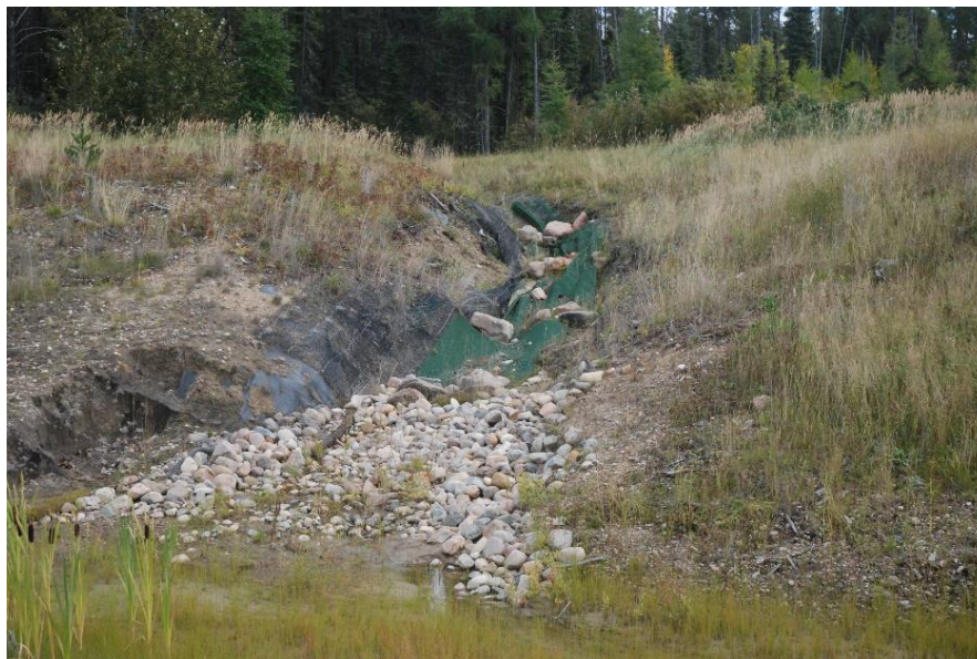
Figure B-4 Erosion control mat installed along southeast slope and water has begun eroding under the mats.
