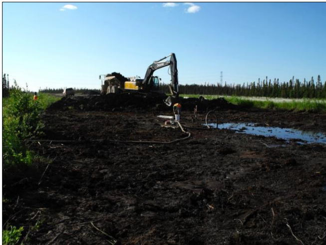
Figure 6: Example of road removal, also showing water management.
