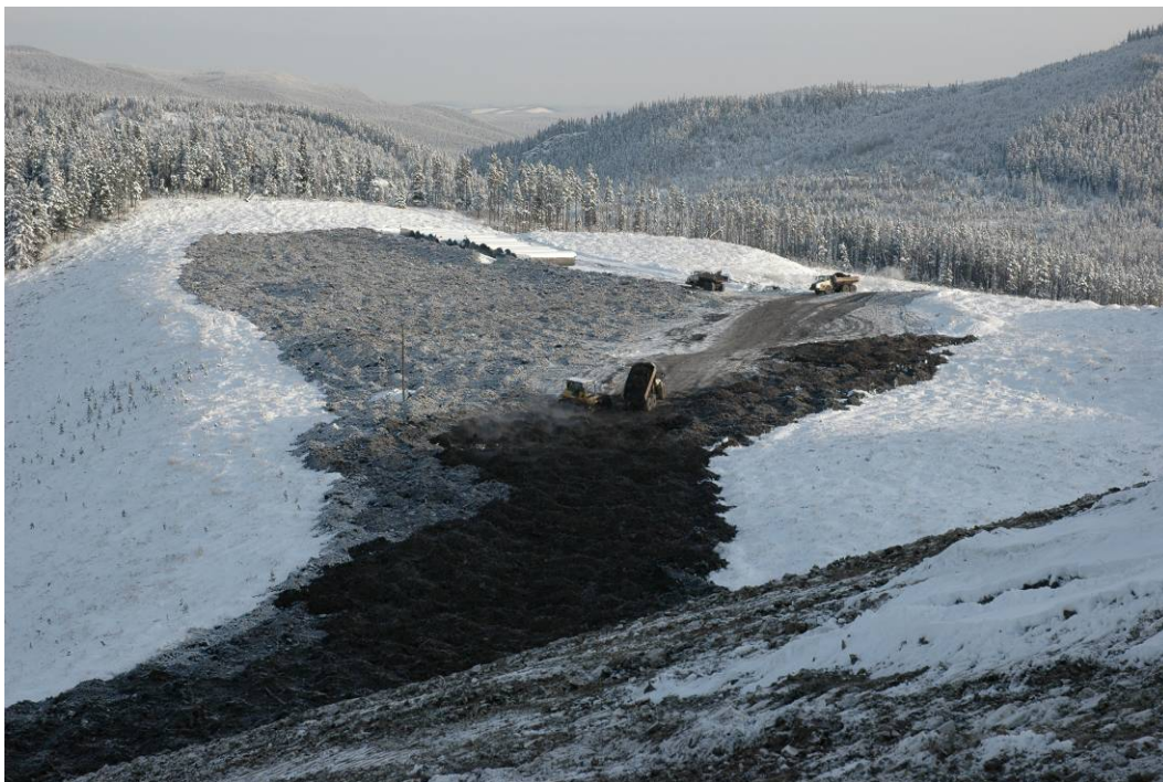
Plate 3.12. Rough/mounded method for soil placement. Photo courtesy of M. Symbaluk, Elk River Coal.
