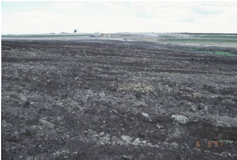
Plate 2.19. After disking peat mix into secondary material at Syncrude Canada Ltd.
