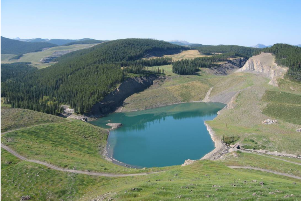
Plate 3.13. Final rough/mounded surface. Photo courtesy of M. Symbaluk, Elk River Coal.
