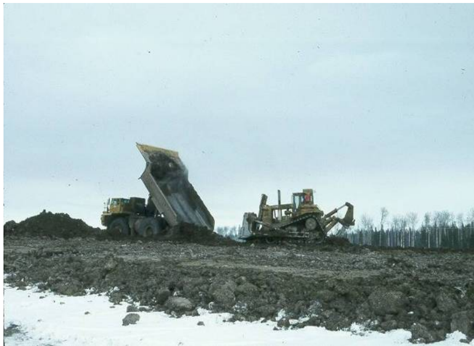
Plate 2.22. Winter soil placement at Syncrude Canada Ltd.
