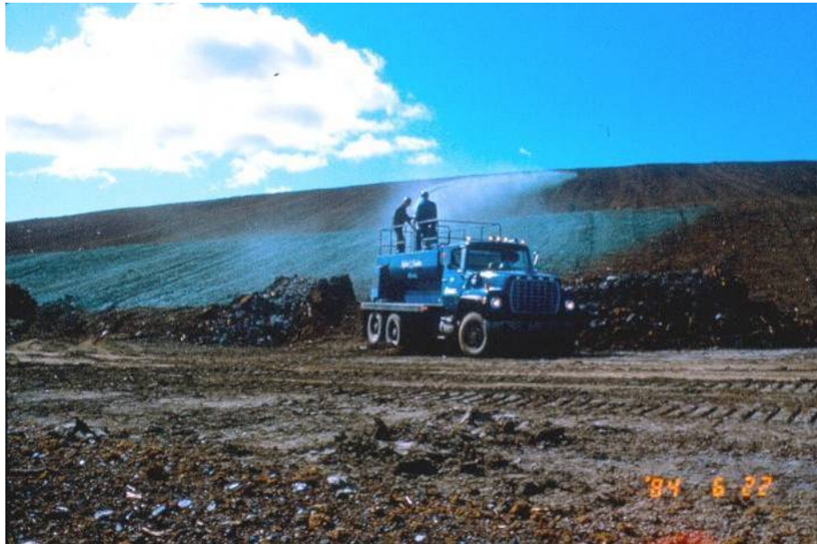
Plate 2.29. Hydroseeding at Suncor Energy Inc.
