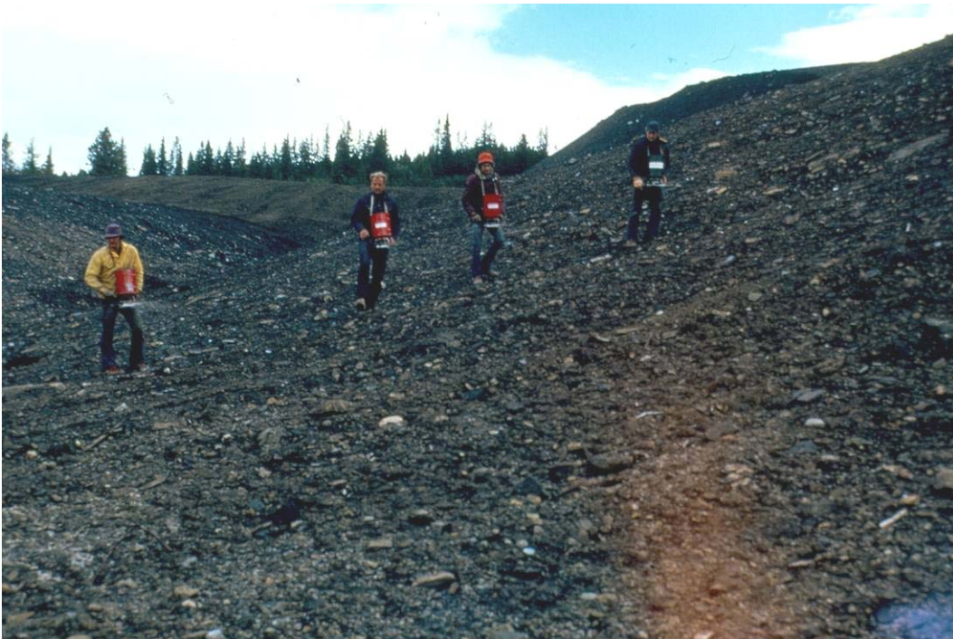
Plate 3.30. Hand broadcasting seed and fertilizer.
