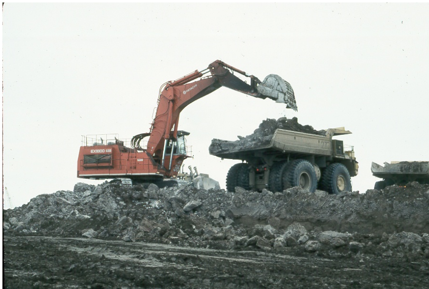
Plate 2.4. Soil salvage operations at Syncrude Canada Ltd.
