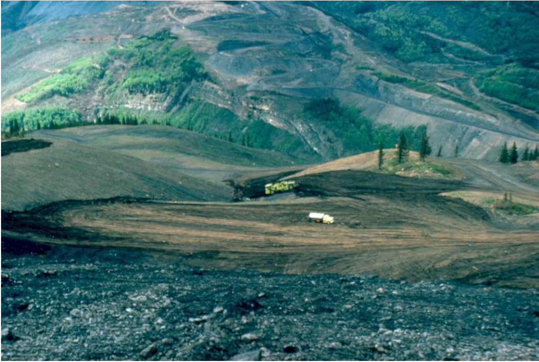
Plate 3.14. Scrapers were used to spread soil in more gently sloping areas.
