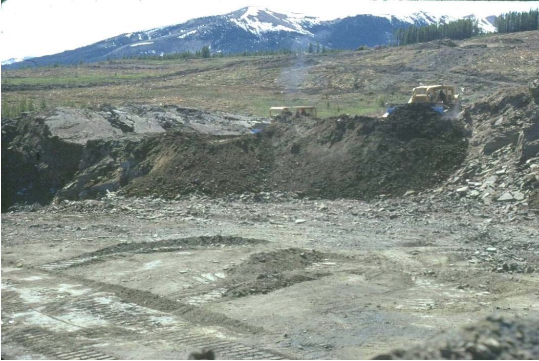
Plate 3.7. Soil salvage in one lift.
