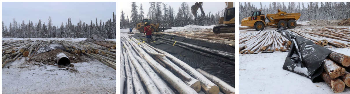
Figure 2: Pre-embedded solid steel culvert covered with mineral fill and abutted with logs. Centre: HDPE pipe bundle being installed among corduroy logs. Right: Log bundle wrapped in a geotextile placed among corduroy logs.
