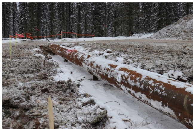
Figure 1: Culvert resting on piles at target embedment elevation. A trench was dug prior to installing the piles so that the culvert's elevation could be set to the desired post-construction embedment elevation. Right: Saddle design detail. (Drawing produced by All-Can Engineering & Surveys (1976) Ltd.)
