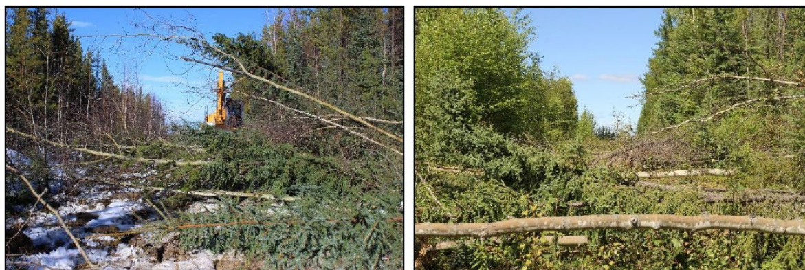
Figure 3: Upland jack pine site treated with a tow-behind Shark Fin Drum with woody materials applied via a Nodwell excavator. Directly after treatment (left) and three years after treatment (right).
