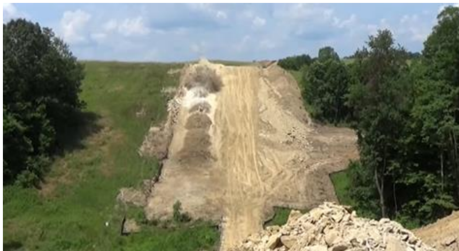
Figure 14. Example of explosives being used to reduce excavation time for a pipeline right-of-way (left side of image). Source: Dykon Blasting.
