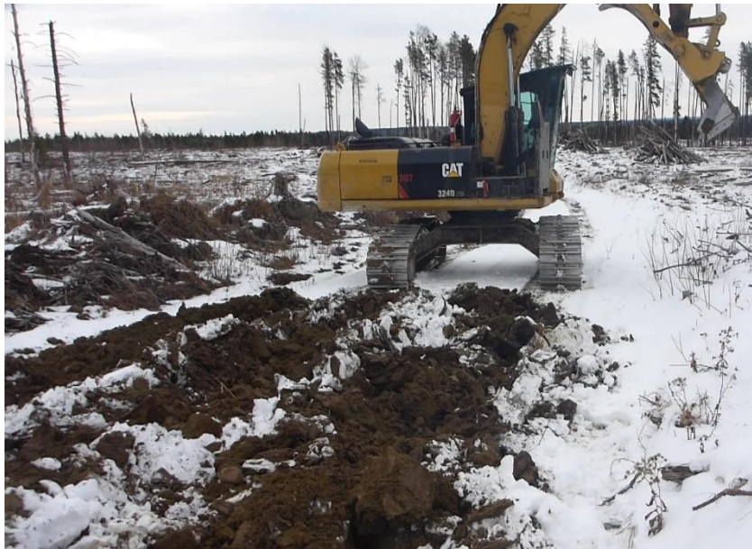
Figure 7. The Excavator RipPlow attached to the arm of an excavator and being used to decommission a forestry road.
