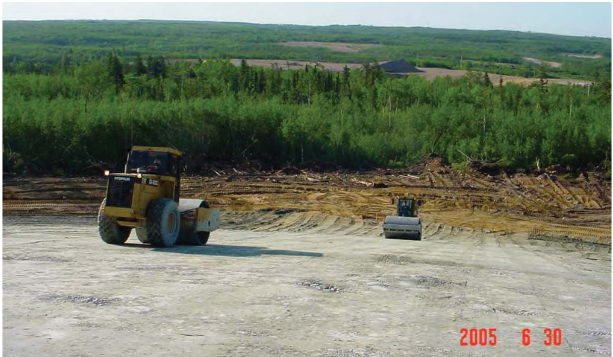
Figure 2. Photo of the re-graded Claude WRP being compacted in 2005 prior to till cover placement.
