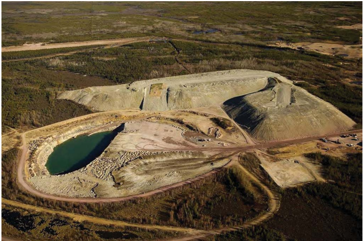
Figure 1. Photo of the Claude waste rock pile in about 2003 prior to pile re-grading and cover system construction (Claude pit being backfilled in the foreground).
