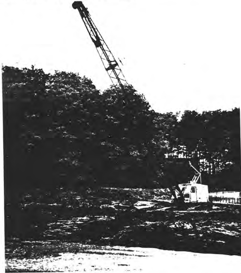
FIGURE 2: THE DRAG LINE AND SPOIL PILES, 1979
