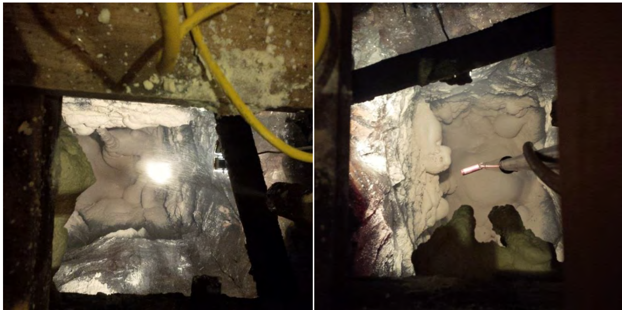
Figure 8: Application of Polyurethane Foam Plug and Cavity Monitoring Survey Using the C-ALS System
