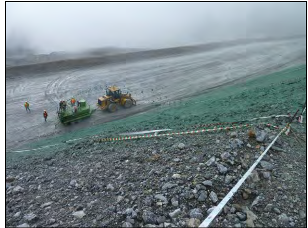
Figure 10 – Application of slurry to top of slope
