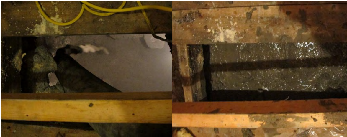
Figure 11: Pumping specified 25 MPa concrete for final plug
