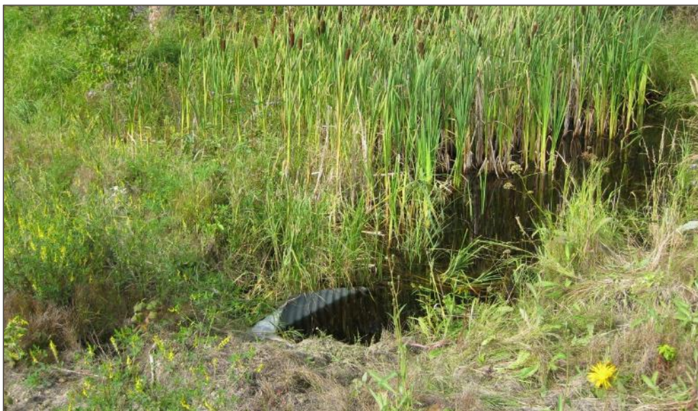
Figure 15. An example crossing where concentrated flow has created flow channels at the exit point of the culverts, even though multiple culverts were used. Photo courtesy of FPIInnovations.
