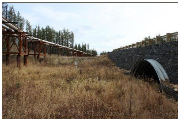
Figure 22. A geosynthetic reinforced soil (GRS) arch used as an alternative to a bridge over a defined water course (left) and a pile supported GRS jump span bridge crossing a sensitive wetland habitat.
