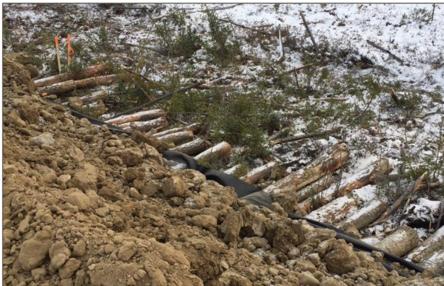
Figure 27. Corduroy placement on an in-situ oil sands road, with a geotextile separation layer on top of the corduroy logs.
