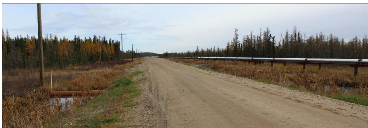
Figure 14. Example of a road where culverts were only placed at topographic lows, resulting in this 500-m stretch of road with a single culvert. Dead trees and trees with reduced vigour were observed beside the road on the ponded side; trees showing increased vigour are found on the drier side.
