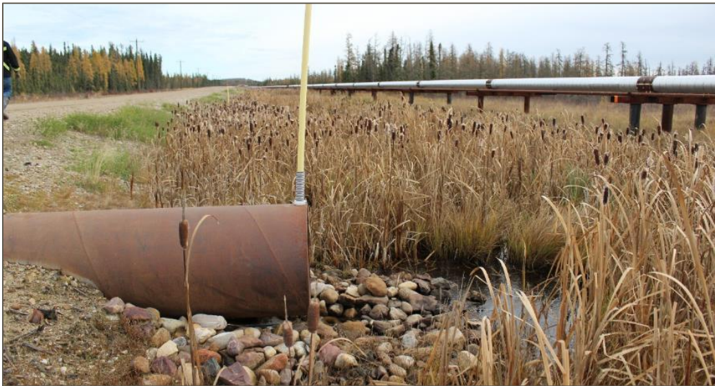
Figure 20. View of a solid steel pipe used as a culvert. Note the pipe is higher than the water surface, indicating the need for precise elevation controls during construction. Partial embedment is a common practice in the forestry sector.
