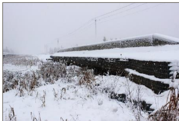
Figure 22. A geosynthetic reinforced soil (GRS) arch used as an alternative to a bridge over a defined water course (left) and a pile supported GRS jump span bridge crossing a sensitive wetland habitat.
