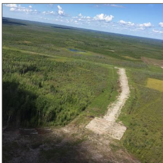
Figure 28. An example of road (left) and pad (right) construction at an in-situ oil sands facility using corduroy as a base foundation.
