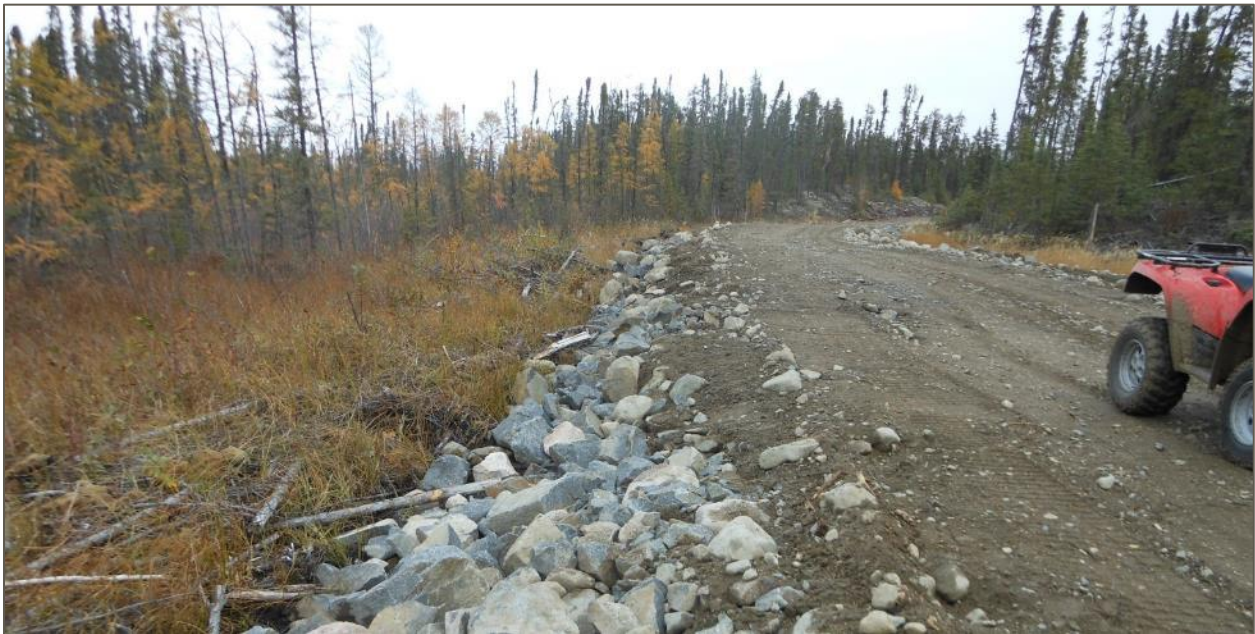
Figure 8. Permeable rock mattress used beneath a resource road in a wetland. Photo courtesy of FPIInnovations.
