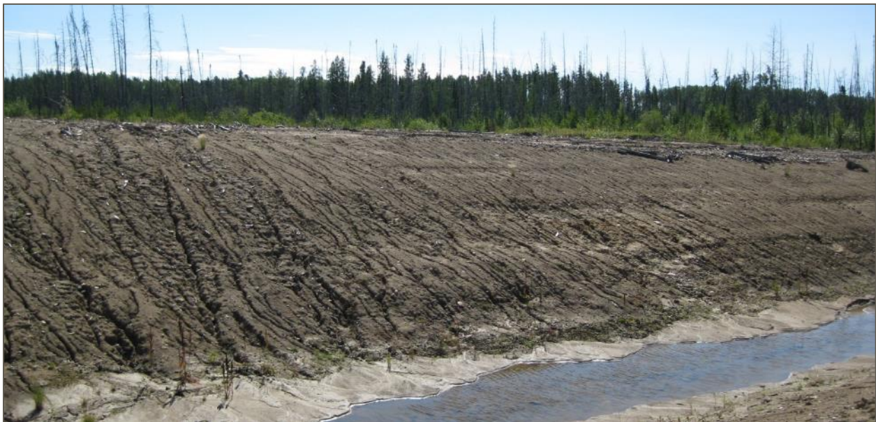
Figure 11. An example of a perimeter berm for an in-situ oil sands pad that would benefit from additional erosion control measures. Photo courtesy of FPIInnovations.
