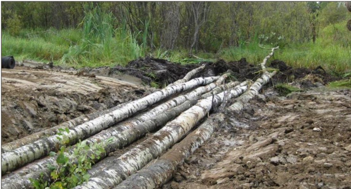
Figure 6. An example of a log bundle used to enable water flow along a long-term forestry road. Photo courtesy FPIInnovations.
