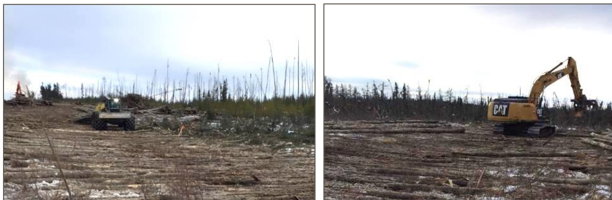
Figure 26. Logs are generally brought to site using a skidder and placed with an excavator.
