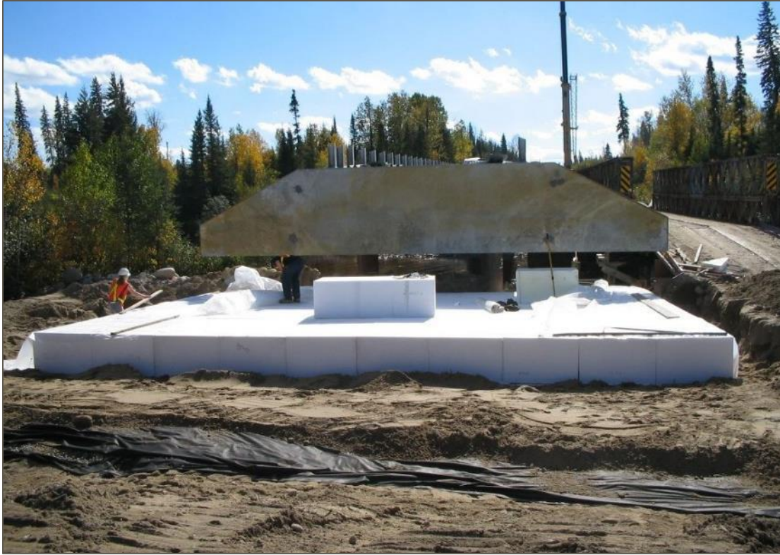
Figure 7. Example of the use of expanded polystyrene showing typical dimensions of the blocks. Note that expanded polystyrene can be used as a lightweight fill as well as for other engineered specifications, such as void forms. Photo courtesy of Tembec.
