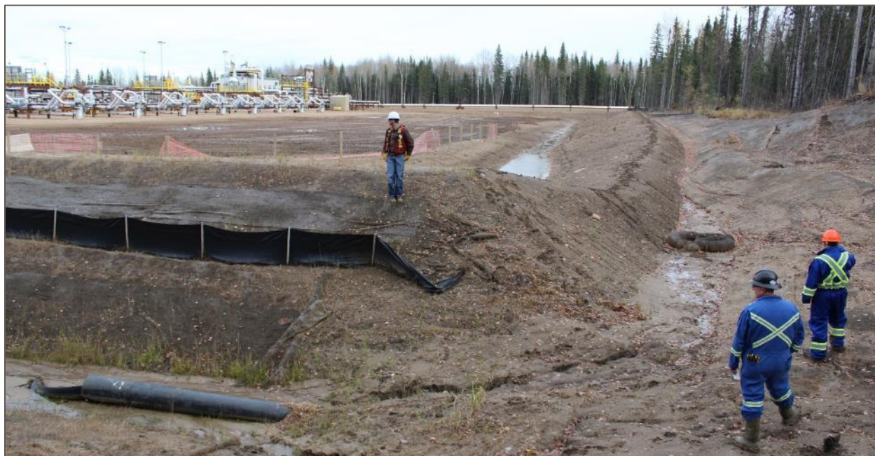
Figure 31. An example of a cut and fill pad with significant groundwater flow and weeping tile installed to divert water from the pad, preventing saturation of the pad base.
