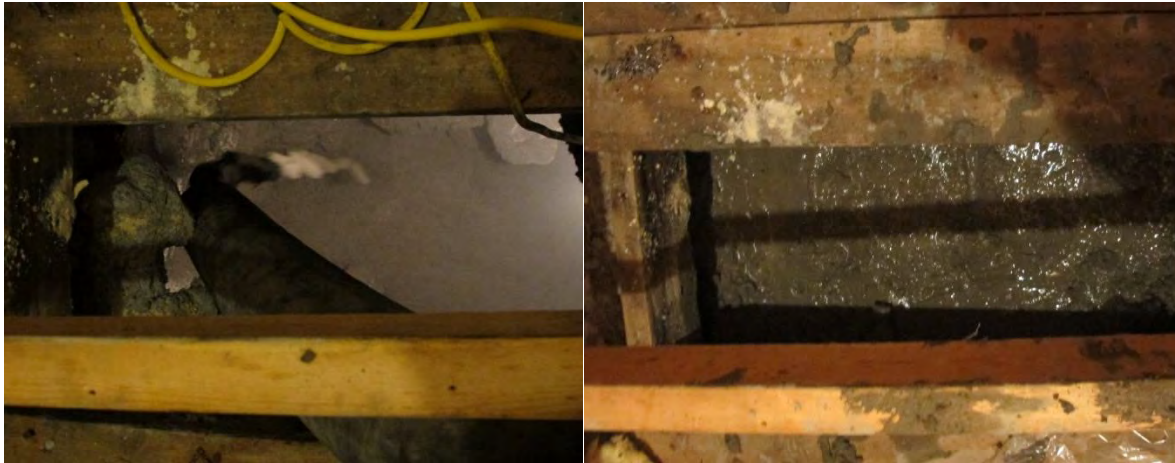
Figure 11: Pumping specified 25 MPa concrete for final plug
