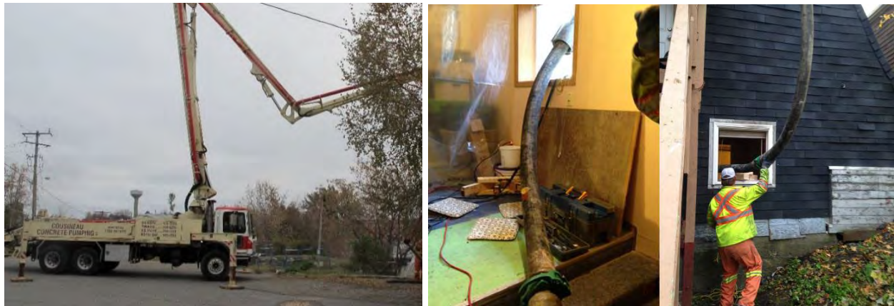
Figure 9: Concrete pump truck and slick line used to pump concrete into shaft void
