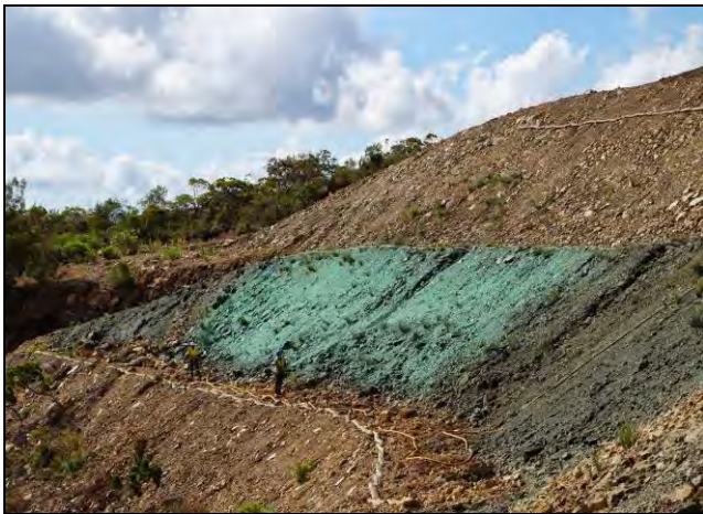
Figure 13 - Second application over compost layer
