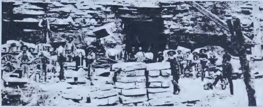
The first mine in Canada at the Forks of the Credit 1886, limestone and sandstone were extracted.
