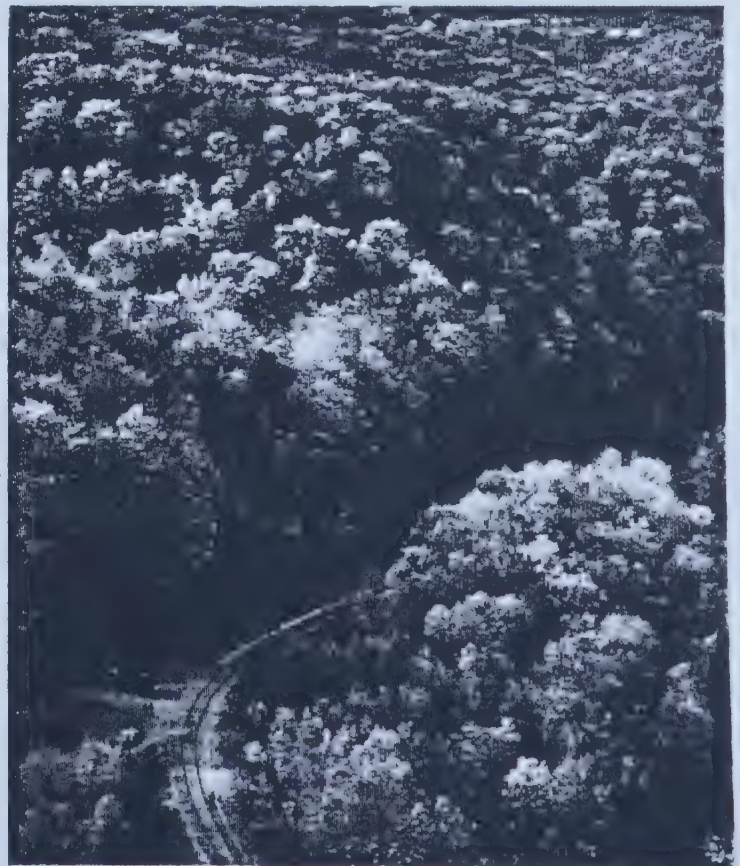
Credit Valley today, looking north to Cataract
